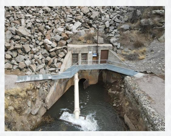
Replaced and extended catwalk located on the dam valve gallery house
