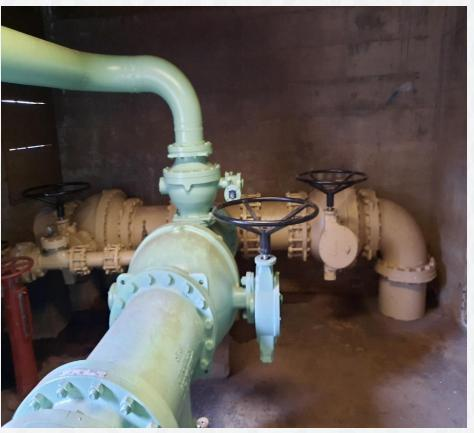
Replaced all valves and piping inside the dam valve gallery
