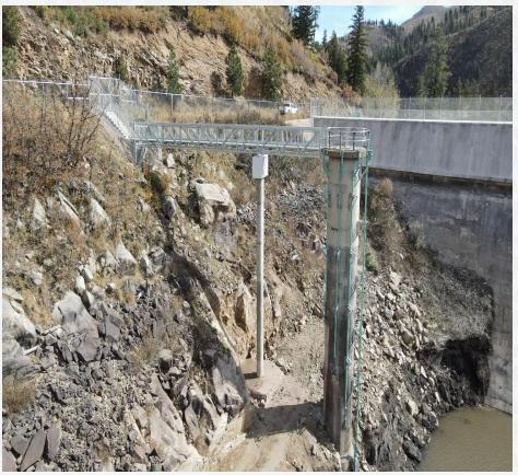
Replaced the existing valve on the intake structure and added three additional intake ports at various levels for improved water quality. Installed a catwalk for operator and maintenance access, thus saving time and improving safety
